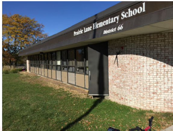
Classroom door propped open for ventilation (security issue typical at several Elementary schools)
