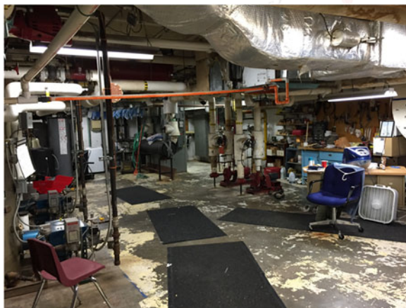
Boiler room - Storm shelter
